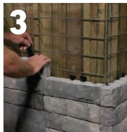
3 Attach Tandem Veneer with Connector
